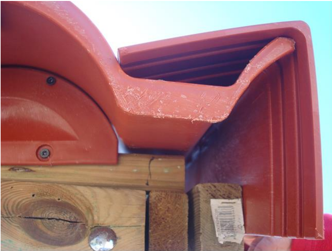
Lateral closure when finishes in canal
