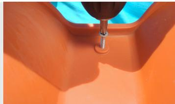
2. The roof is installed from left to right and from bottom to top. It is screwed to the battens on the 4 points marked in each flat channel of the panel.
