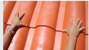
3. The upper row is placed by pushing the panels from bottom to top until male and female parts of the anchorage fit.
